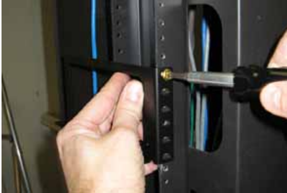
Figure 18: CX II/CXi II Controller Rack-Mount Installation - Attaching Brackets to Rack Frame
